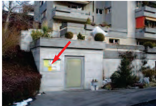
Bürgstrasse Nr. 23, BKW Trafostation
