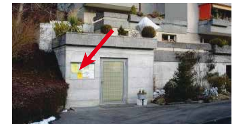
Bürgstrasse Nr. 23, an BKW Trafostation
